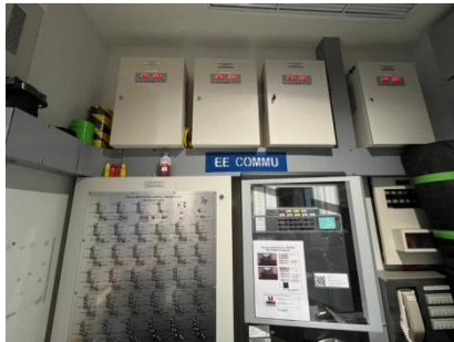
Fire Alarm Control Panel
