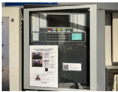
Graphic Annunciator Fire Alarm
